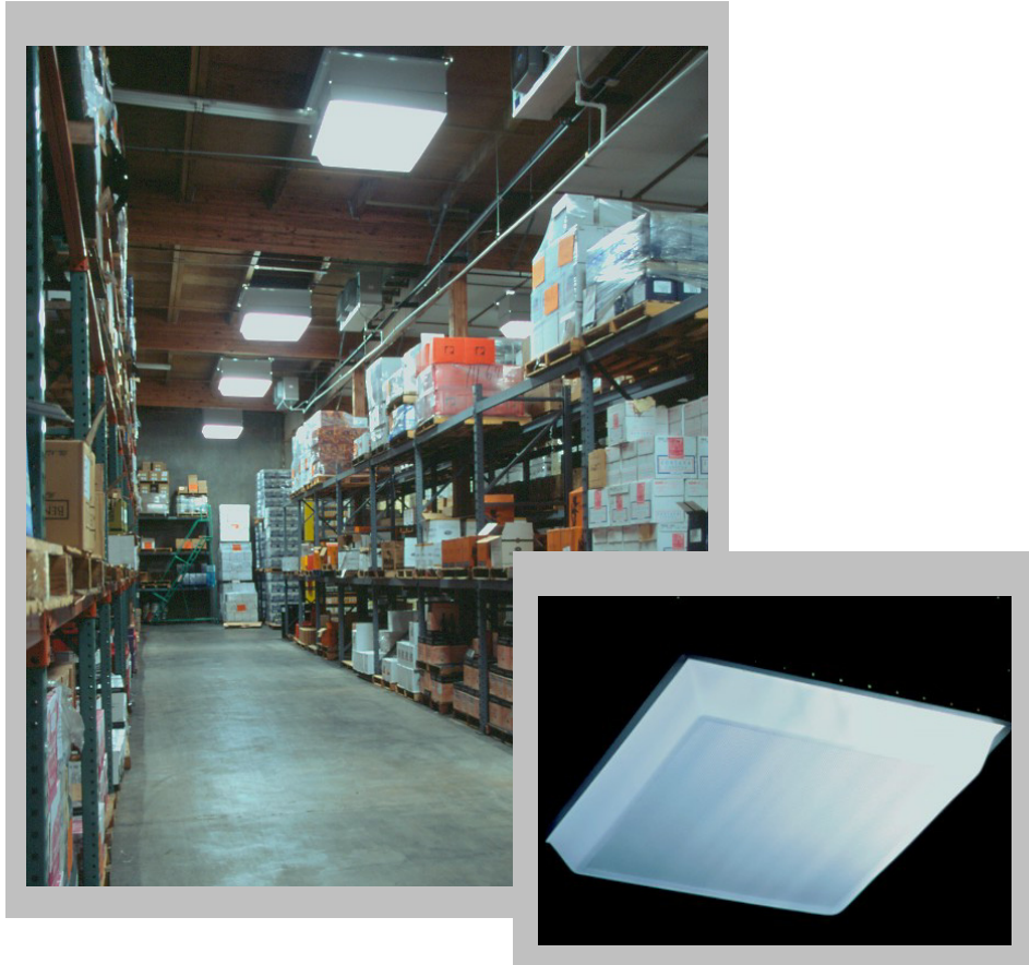
Figure 3-26. Better Brands warehouse, Oahu. Skylights with integrated light wells, fluorescent lighting, and diffusers (inset). Photos: Erik Kolderup, Eley Associates.
